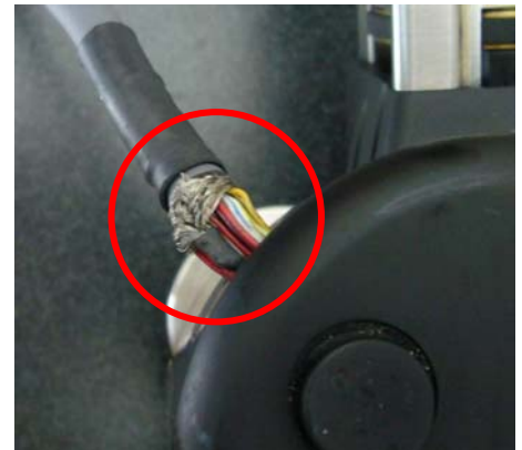
Figure 4.10: Excessive twisting of cable causes damage.
