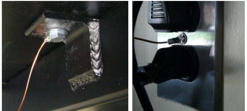
Figure 16.6.3: ground the acoustic hood to wall socket with piece of copper wire.
